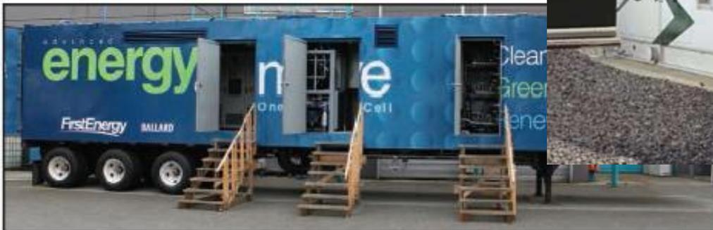
(Above) This tractor-trailer-sized generator from Ballard produces 1 MW of additional power using hydrogen fuel cells. FirstEnergy Generation Corp., Ohio, U.S.A., is installing the unit to provide peak power in Eastlake, Ohio, for a five-year trial. (Right) The fuel cell system comprises nine modified bus fuel cell modules arranged in three banks of three.
